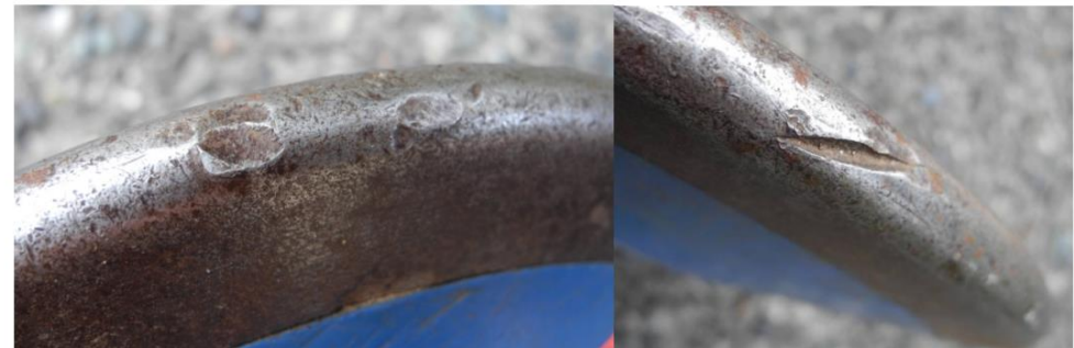
The above cracks and dents can be repaired, and therefore are not level. But service
